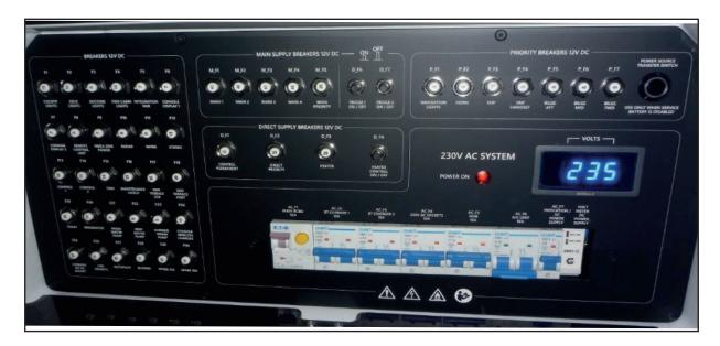
12V DC circuit breakers and 230 V panel board
